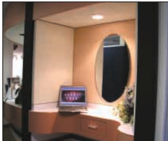
Fig. 6 Stand-up consultation room in Dr. David Hamula's office, with custom-fitted Victratex acoustical panels, covered by cloth surface with small holes that allow sound to penetrate.
