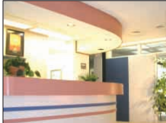
Fig. 3 Front desk with acoustical soffit and panel treatment in office of Dr. David Hamula, Colorado Springs, CO.
